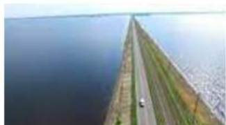
the longest dam in Ukraine
